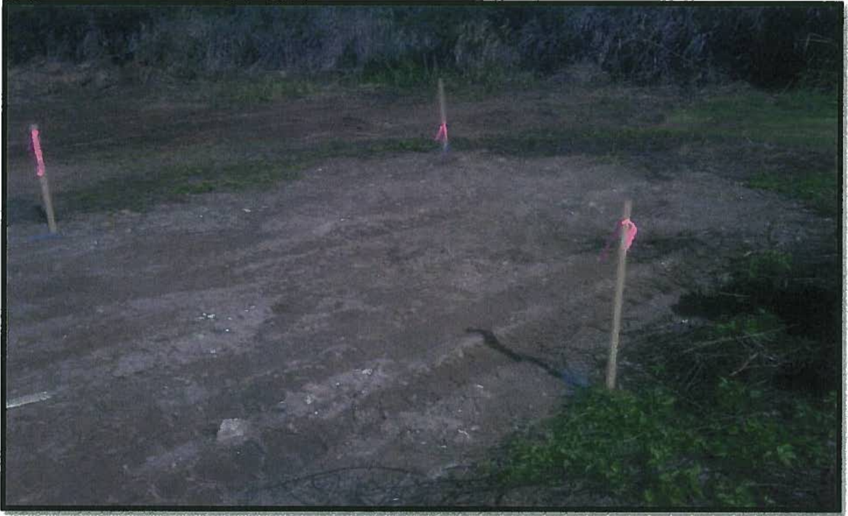
Photo 1. Steel Rack Storage Area after Surface Soil was Removed.
