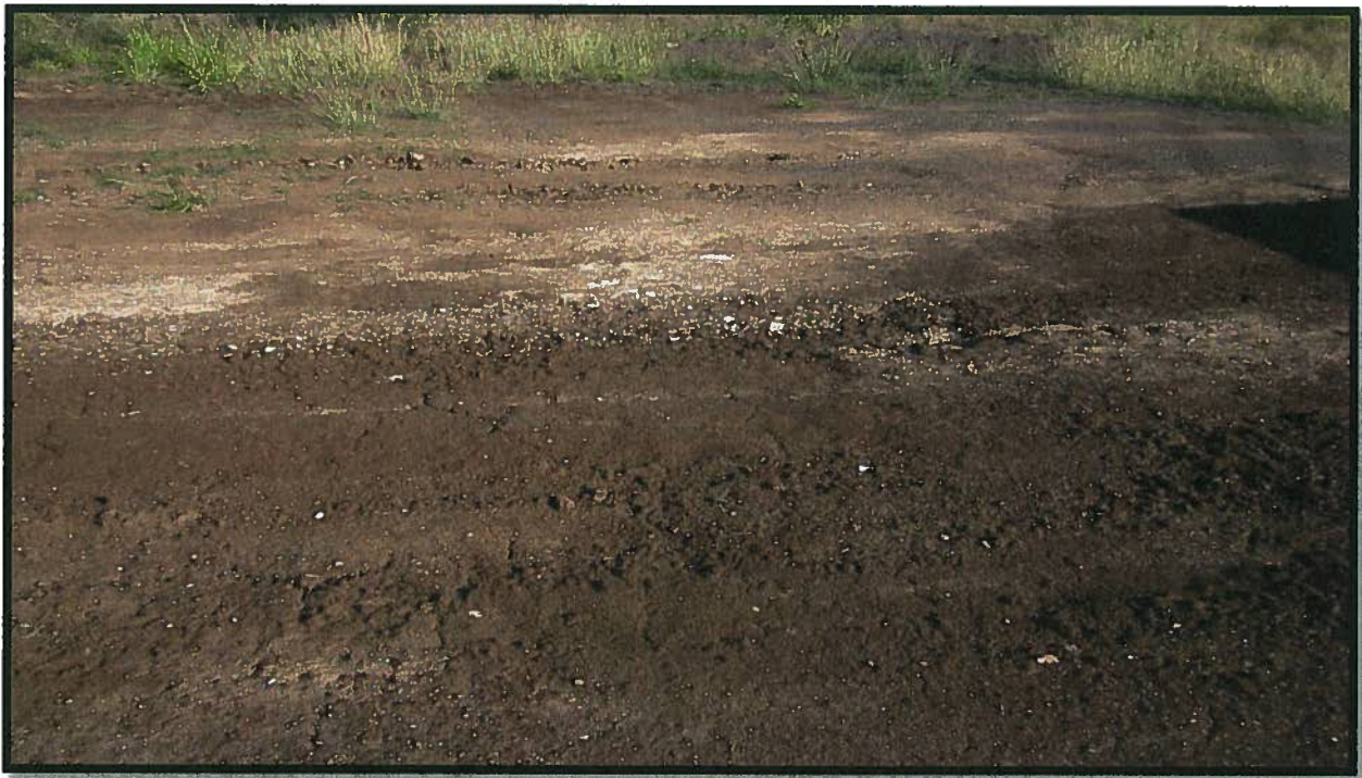
Photo 4. Gas (Fuel) Storage Tank Area after Second Excavation
