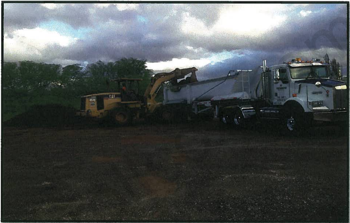
Photo 12. Loading Contaminated Soil into a Semi End Dump
