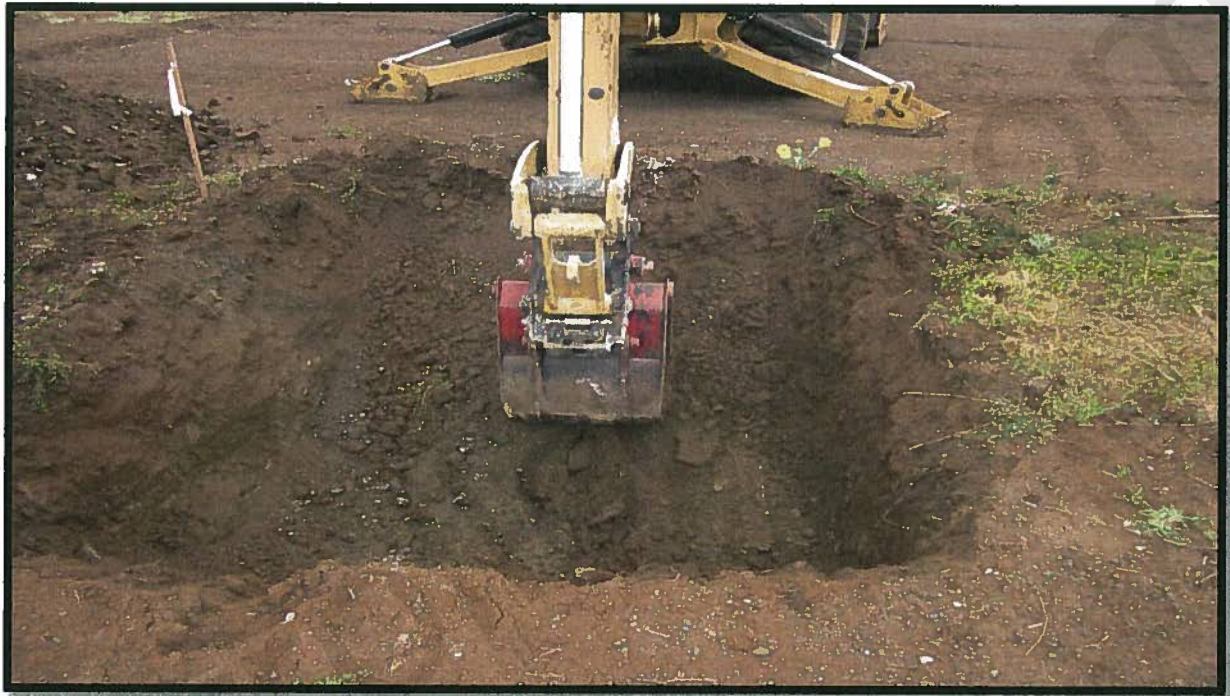
Photo 8. Excavating Contaminated Soil at the Oil Spill Area.
