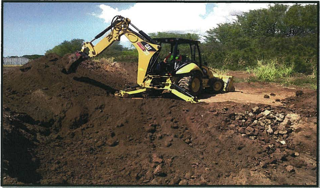
Photo 5 Third Excavation on the Gas (Fuel) Storage Tank Area
