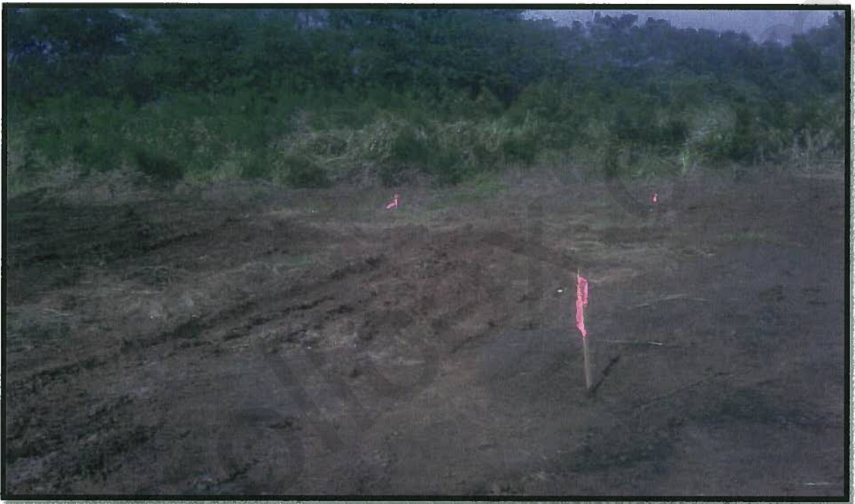
Photo 2. Gas (Fuel) Storage Tank Area After Surface Soil was Removed.
