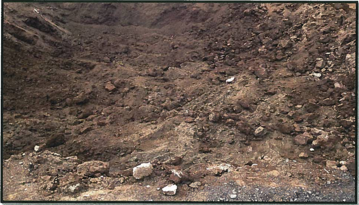
Photo 7. Gas (Fuel) Tank Excavation Area
