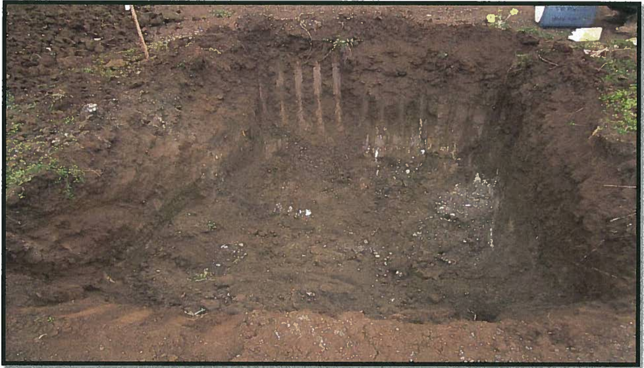
Photo 9. Excavation Pit of the Oil Spill Area.
