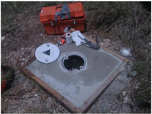
Photograph 6: Completed installation of monitoring well MW-5.
